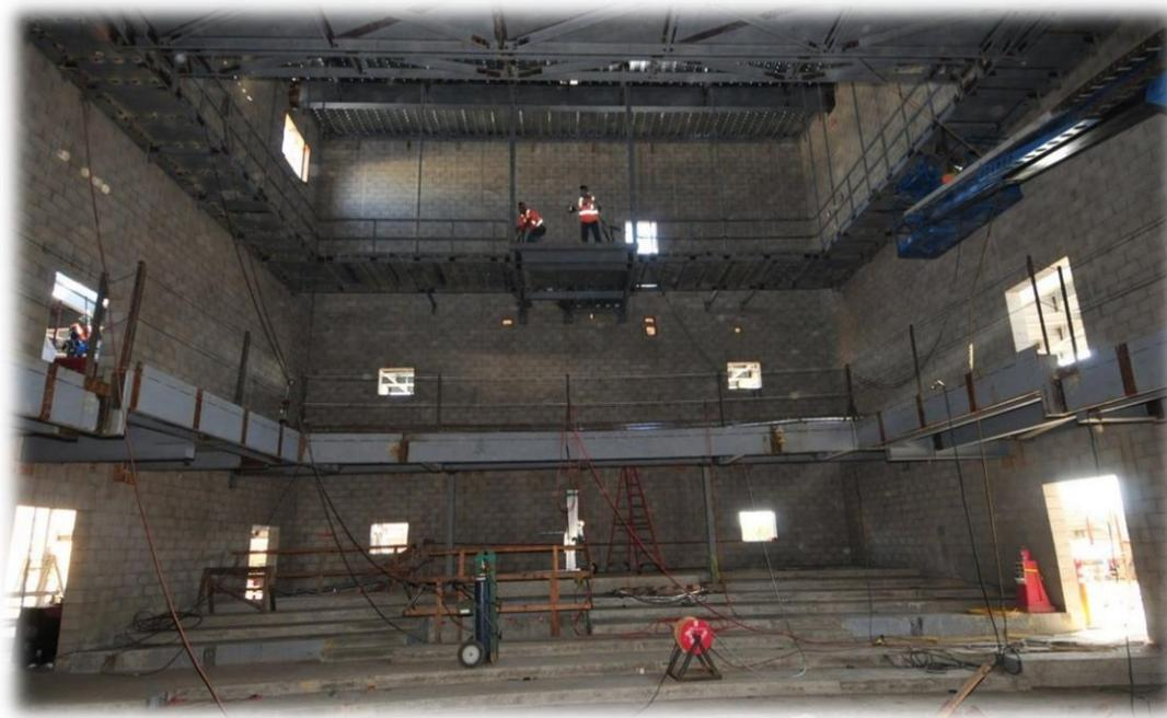
The Performing and Visual Arts Center at Grossmont College will include a new 390-seat theater, with a professional performance stage, orchestra pit and balcony. **Update:** The building's roof is poured in and seating work platform is complete. Ongoing work includes welding the stage grid iron, framing on the west elevation, and grouting throughout the building. In addition, waterproofing efforts are underway.
