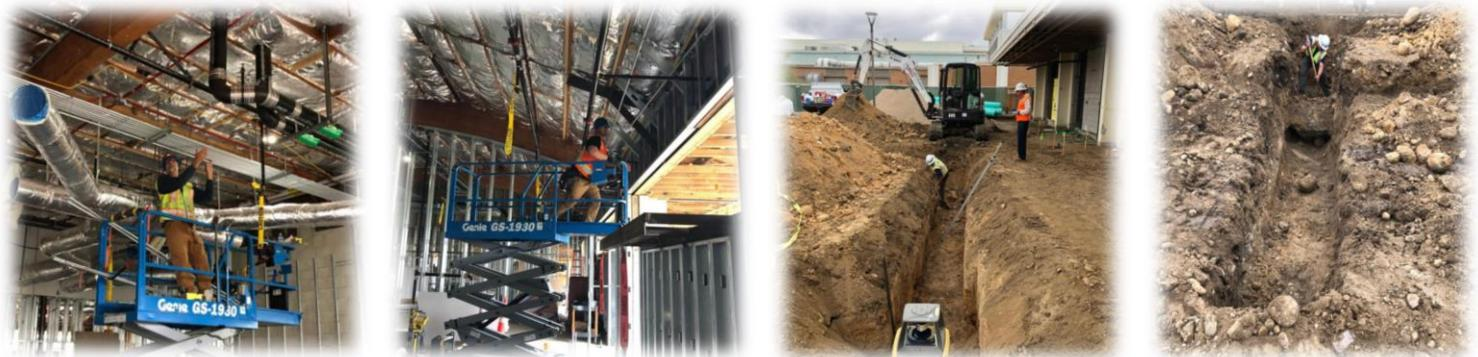
The first phase of the Science, Math & Career Tech complex is the renovation of Building 31. Tenants of Building 31 are housed in the interim swing space located in Parking Lot No. 5 South. **Update:** The 12kv east utility tie-in and storm drain installation are near completion. Framing, tie-backs and steel welding are ongoing.
