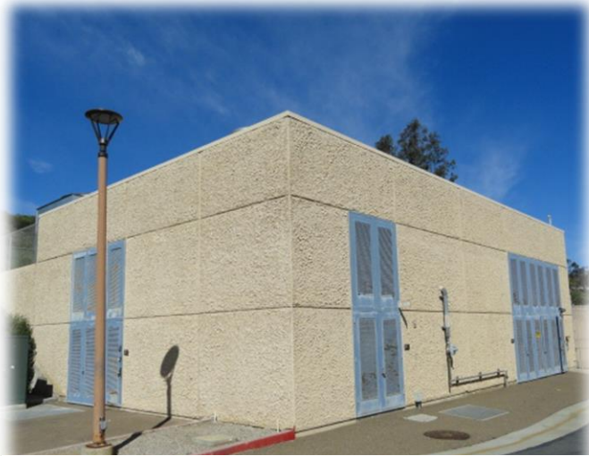
Existing Chiller Plant
